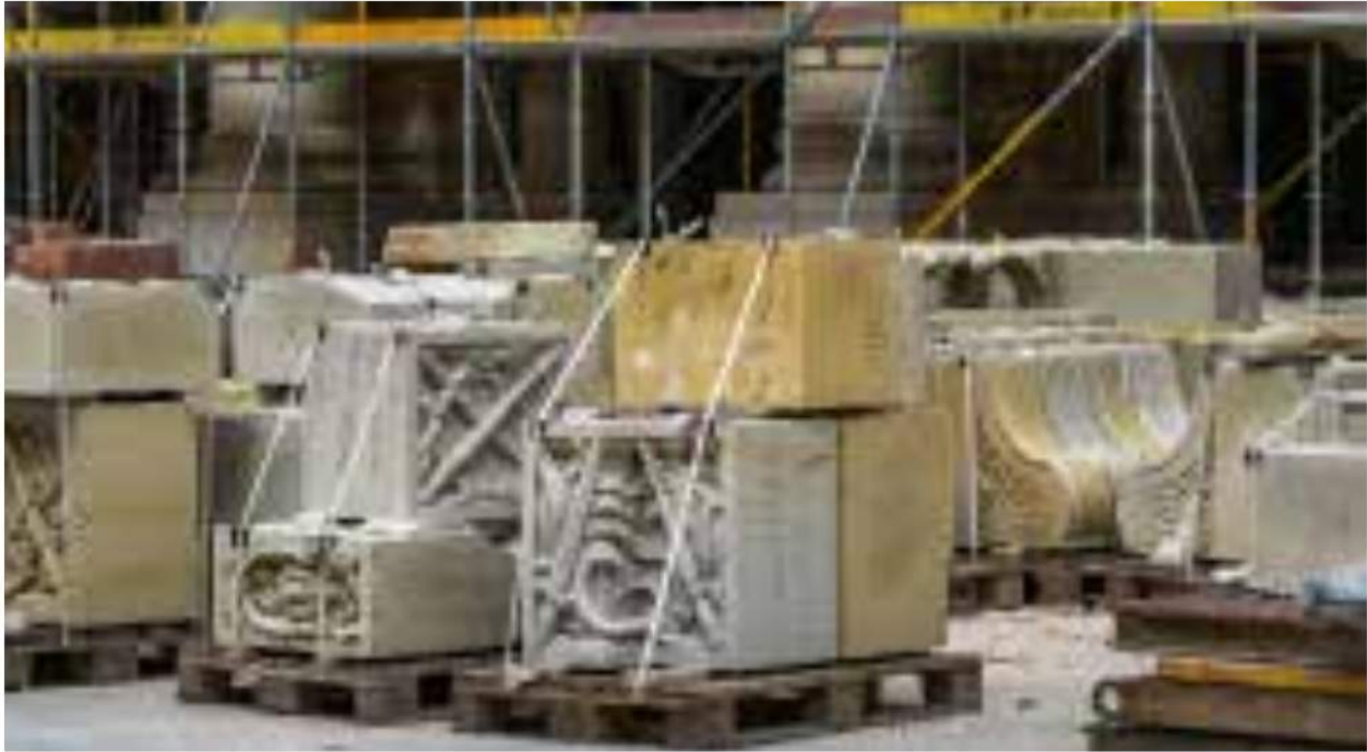
Some decorative elements in the Schlüterhof Court that are about to be integrated into the façade. © Frank Burchert
